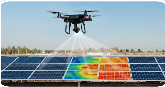
Drone Solar Inspection for Quick Solar Panel Fault Detection
